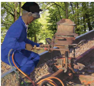
Figure 3.11 Thermit process for joining railway tracks
