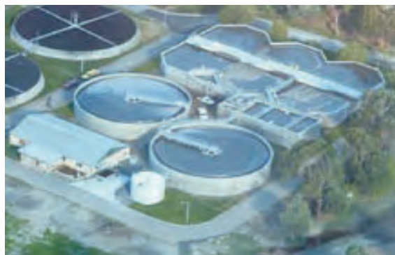
Figure 10.7 An aerial view of a sewage plant
